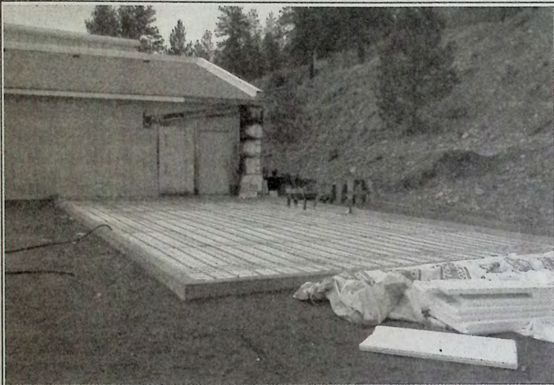
Work continues on the Posse Training Facility at Princeton Arena. *
