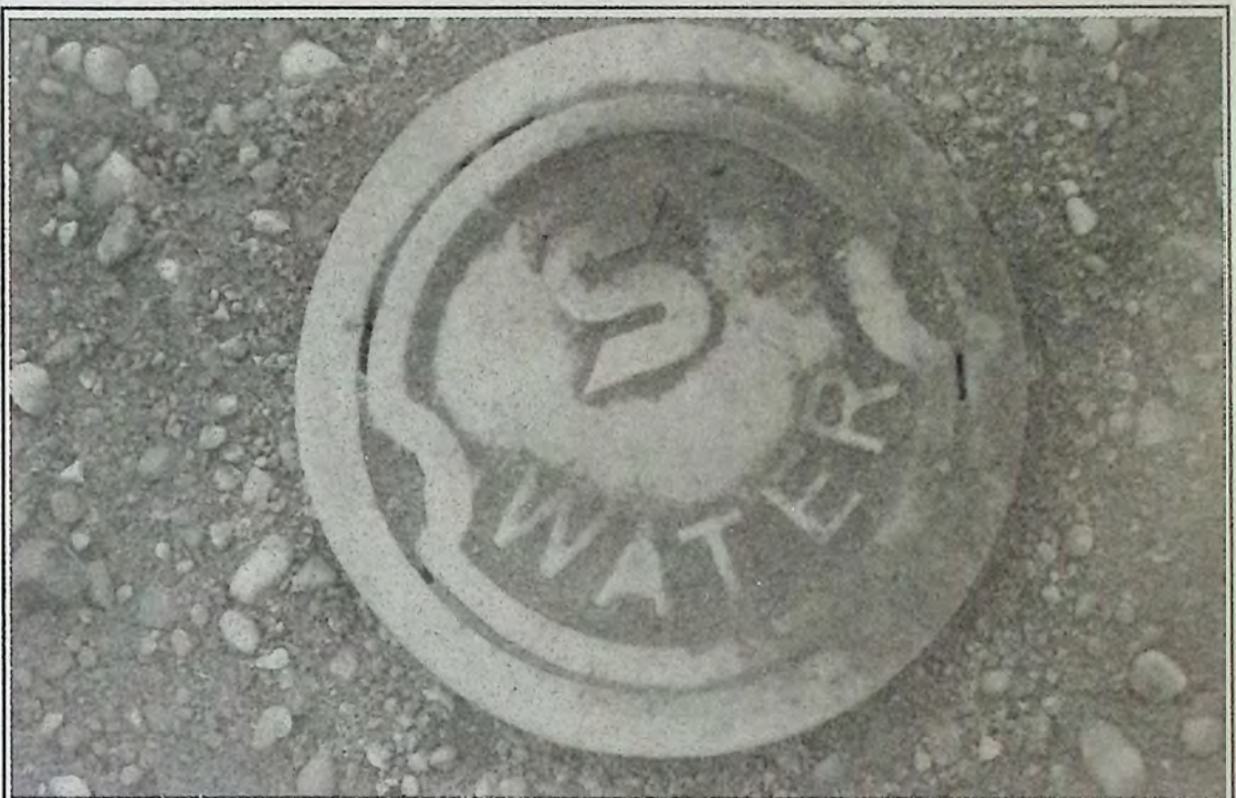
Proof water lines are in the industrial park. *
