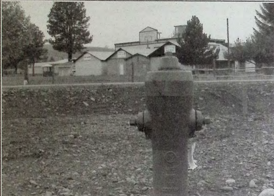
A fire hydrant now sits across from Sunflower Downs - part of the industrial park water project. *
