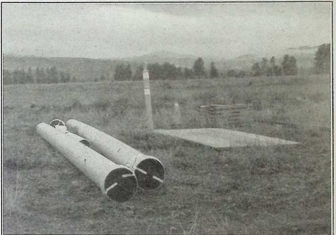
Signs of progress from the East Princeton Water Project. *
