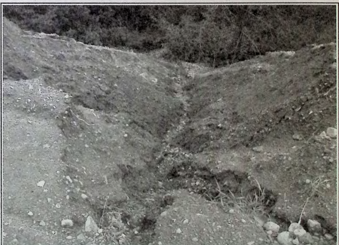
Looking down one of the washouts along Tulameen Road. Photo: Brenda Engel
