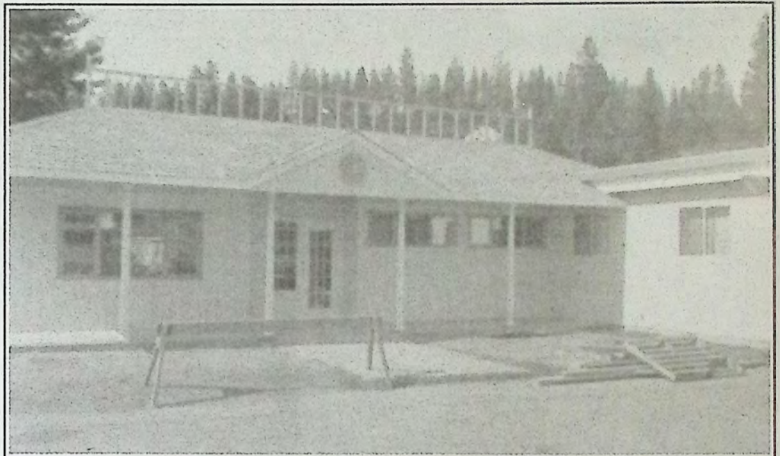
The public health building as it looked in 1987 during revitalization. Photo: Dawn Johnson
