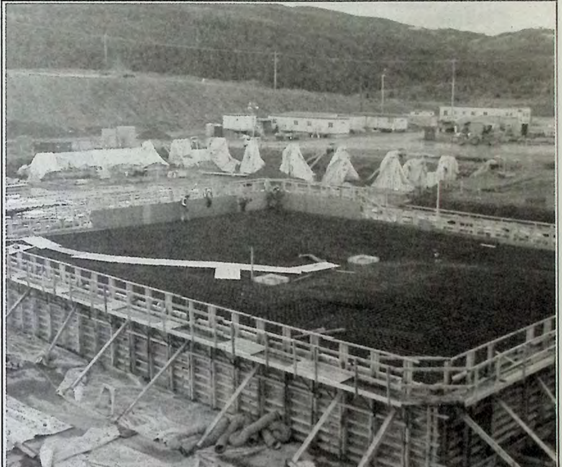
The new SAG Mill rebar and forms at Copper Mountain. Photo: CMMC
