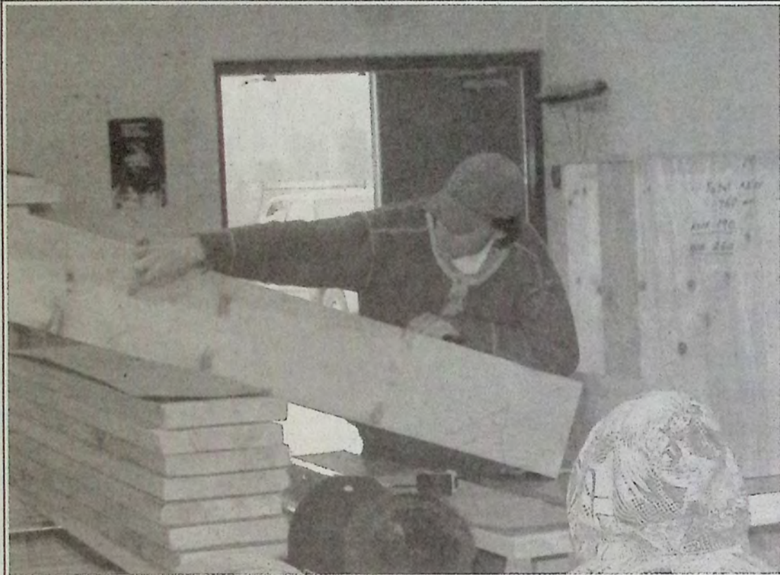
The math involved in building a set of stairs/steps was explained March 2 as part of the Yes 2 It Program presented to Grade 8 students at Princeton Secondary School. *
