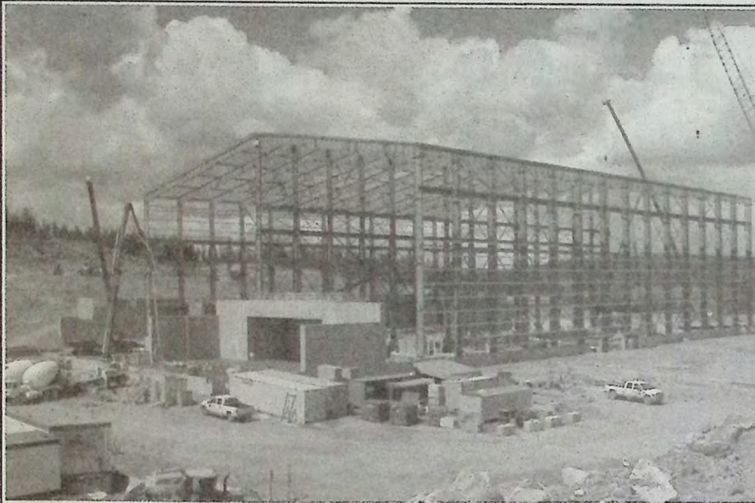
The concentrator building construction is on schedule at Copper Mountain Mine. *
