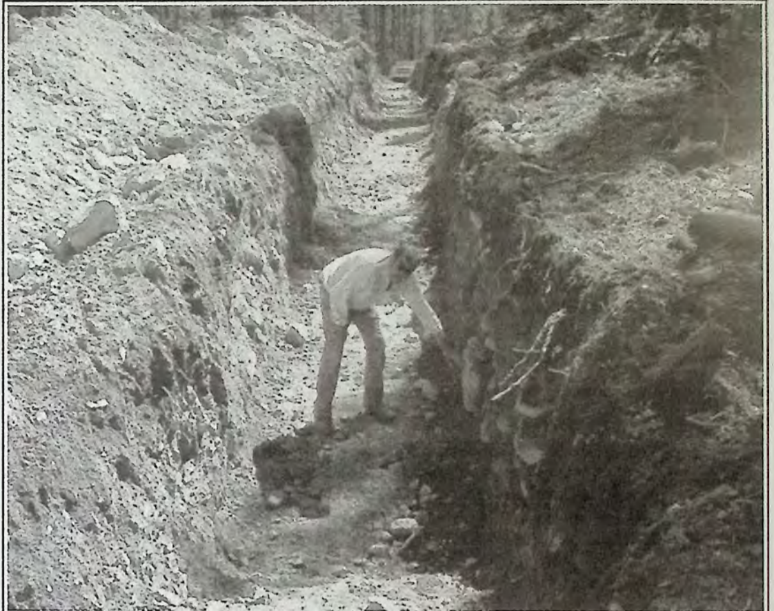
Geologist Leonard W. Saleken inspects trenching work. Photo: Goldcliff Resource Corporation.
