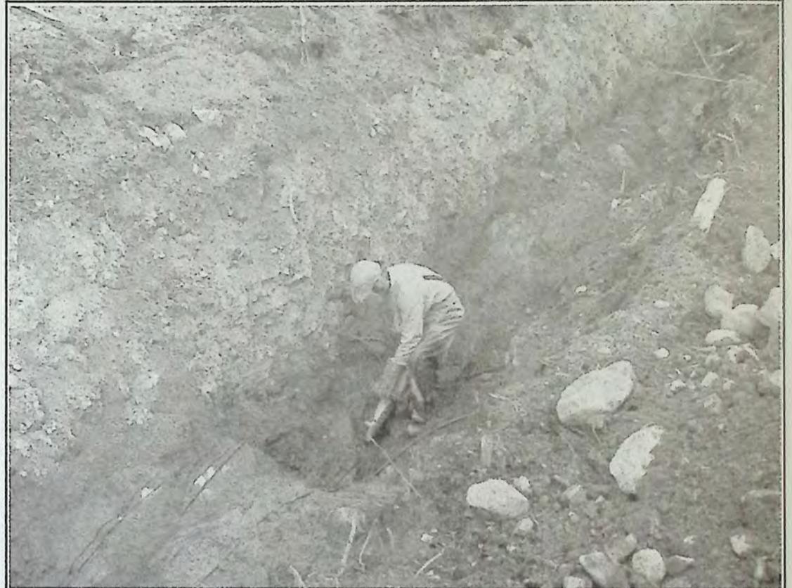
Trench sample cutting on Goldcliff property near Hedley, BC. Photo: Goldcliff Resources
