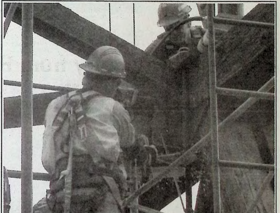
A close-up view of one of the metal rods being cut for removal and replacement. This rod is being cut near the top of the wooden bridge with another cut to follow. *
