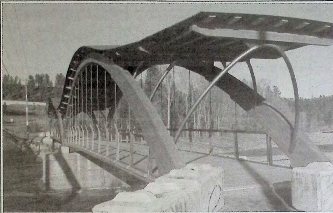
The Bridge of Dreams as it looked a year ago. It was finished in late November of 2009. *
