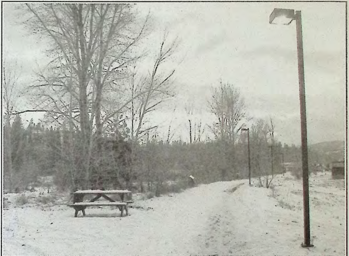
Lights now follow the Trans-Canada Trail along the Similkameen River and down to the tunnel under Highway 3. The lights were turned on December 8th by electrical contractor Hayes Creek Electric. *
