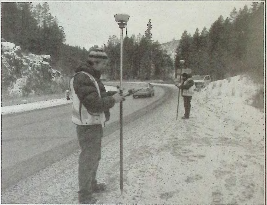
Francois Chabot and Ron Deo of R.F. Binnie Engineering in Burnaby are pictured mapping the road surface and roadbed depth just east of Yellow Lake on December 1st. Photo: Arlene Arlow
