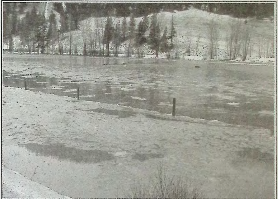
Another view of the flooding caused last week along Highway 3. Photo: Brenda Engel
