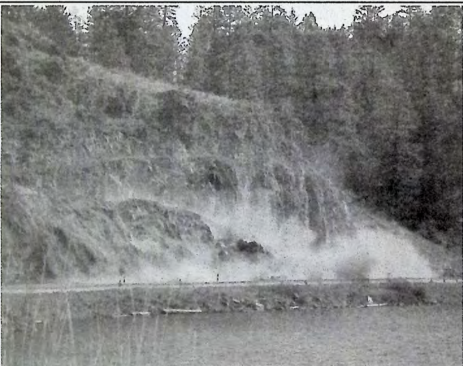
Dust fills the air after the displaced rock settles back down to earth. Notice that the bulk of the dust has been pushed "out" where the blast mats were placed. Photo: Arlene Arlow
