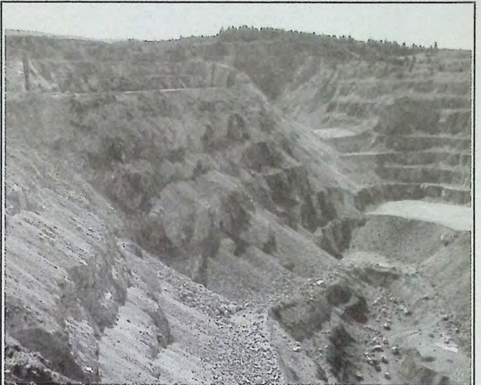
The walls of the pits are 18-metres high. A second pit is in the background. *
