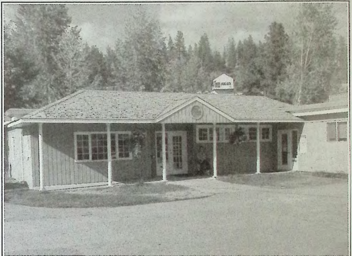
Princeton Community Services building located at 47 Harold Avenue, (corner of Harold and Lime Street), next to Rotary Park along Tulameen River. Photo: Brenda Engel
