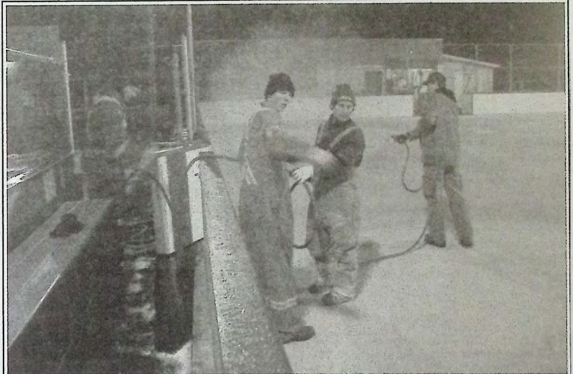
Terry Zeller (second from right) has been putting in volunteer time at the Keremeos Rec Centre outdoor rink for 21 years. The evening of November 29th, he was busy passing on his skills to Tyrell Sladen (far left), Joe Cottrill, and Keith Erickson. The recent warm windy weather had postponed their efforts. Rink prep involves a 1/4 inch of ice base on the concrete subfloor, a layer of whitener, another 1/4 inch of ice followed by painting the lines, and a final 1/4 inch to 1/2-inch layer of ice. Cooling tubes 4 inches apart embedded in the concrete subfloor keep the ice frozen even when the temperature is above zero. The rink should be ready for skating early this week. Photo: Arlene Arlow
