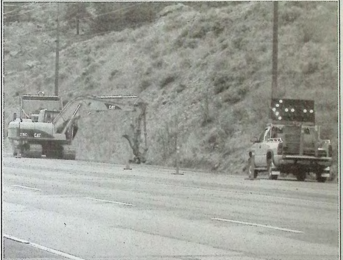
Argo Road Maintenance crews were busy ditch digging along Highway 3 west of Keremeos on February 13th. Keeping highway ditches free of rock debris due to sluffing is a year-long job. Photo: Arlene Arlow
