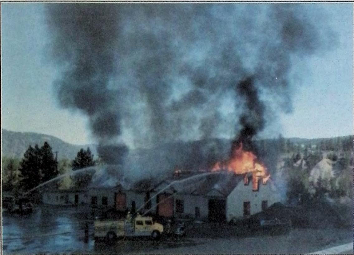
Smoke filled the air in the afternoon of May 11th with a fire at the former Argo Road Maintenance building. Crews from Tulameen, Keremeos and other surrounding areas fought the blaze with Princeton Fire Department. Photo: Brenda Engel
