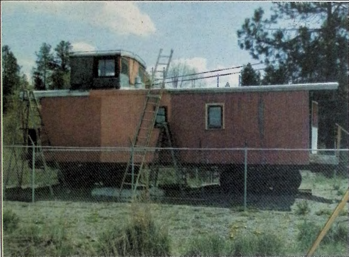
Changes continue to take place at the end of Bridge Street as the old CPR Caboose is restored. Photo: Brenda Engel
