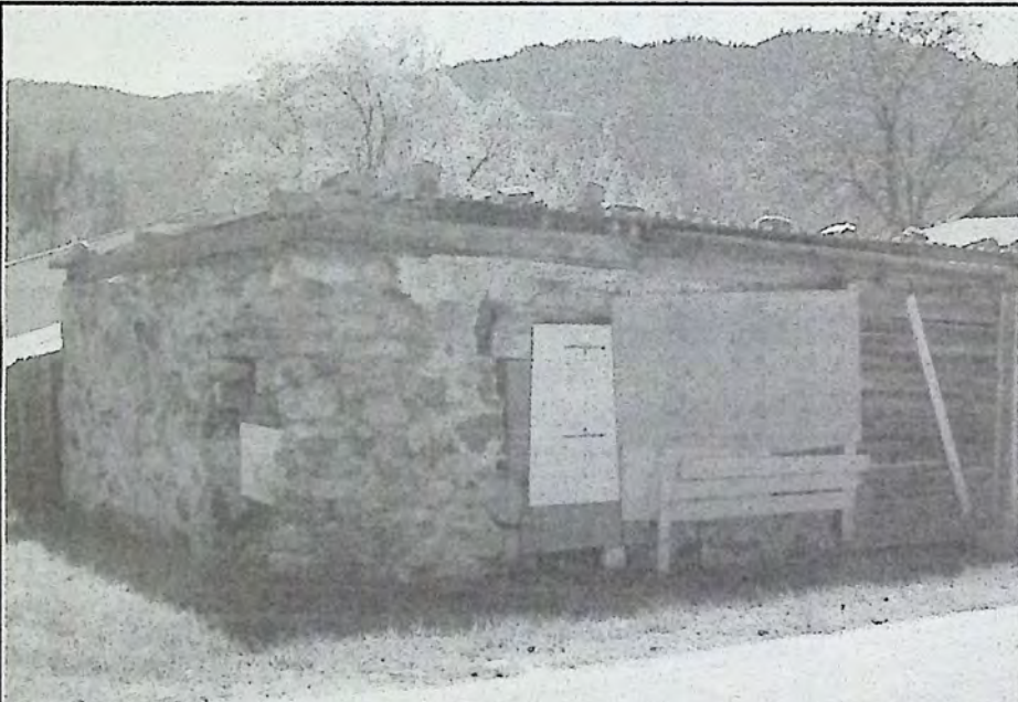
Buildings like this abound in Hedley, remnants of days gone by when manual labour was harder and a days work produced less than today. Undoubtedly the only thing brought in for this structure was the cement and perhaps some shingles: everything else was acquired from the local forest and hills. Families were raised in houses with 3 rooms, sometimes fewer, and houses of over 700 square feet were only for the rich. Imagine! Photo: Arlene Arlow
