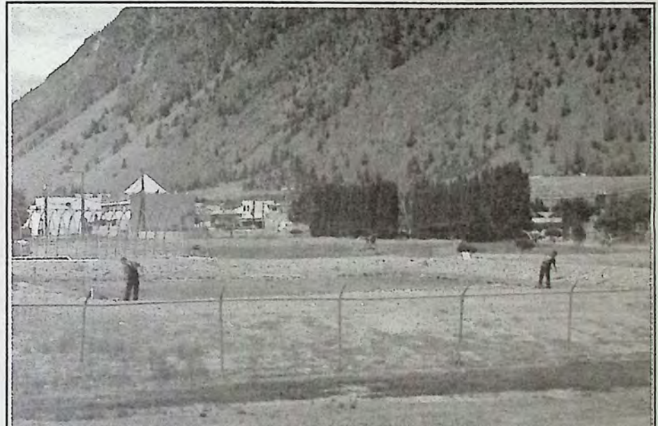
Shae Carlson, left, and Matt Lougheed were busy raking up the biosolids from an infiltration bed at the Keremeos Waste Water Treatment Plant May 24th. The biosolids remain after waste water evaporates and leaches downward into the groundwater. Matt says that the water leached out through natural processes is safe enough to drink! Infiltration beds are each drained and raked as frequently as each month. The biosolids are stored and ultimately trucked to the landfill in Okanagan Falls. Man wells adjacent to the Waste Water Treatment Plant are tested quarterly. Photo: Arlene Arlow
