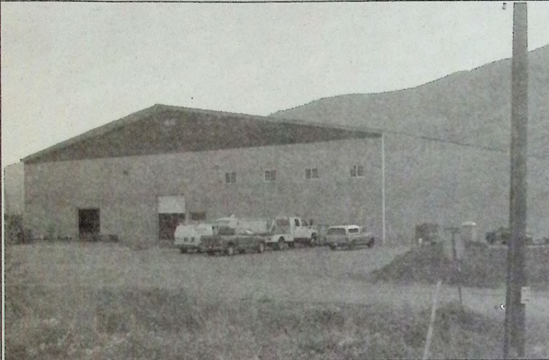
The new cold storage facility in Cawston is coming along nicely. Not all residents were in favour of the facility being built on agricultural land. Efforts of the workers at Cawston Cold Storage Ltd. to unionize were met with some measure of resistance from the employer and were noticed by the British Columbia Labour Board. The BC Labour Board issued a "remedial certification" earlier this year which essentially certifies the union without any red tape. Reasons for the hasty certification included their position that the company "interfered with the organizing drive in such a way that it met the test to issue a remedial certification." Photo: Arlene Arlow
