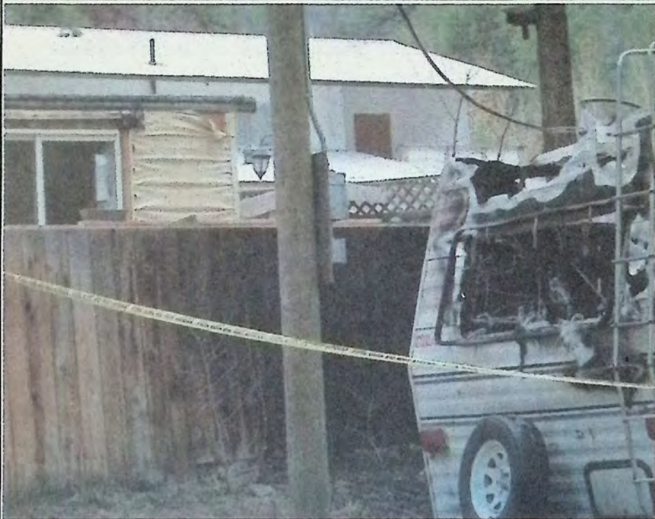
Fire crews credit a 5-foot wooden fence for preventing the spread of a 5th-wheel trailer fire in Olalla last week. Blackened fence can clearly be seen west of (behind) the remains of the trailer. Melted siding on the neighbouring mobile home is visible under the neighbouring home's eaves. The yellow 'Fire line do not cross' tape indicates that the fire is still under investigation. Photo: Arlene Arlow
