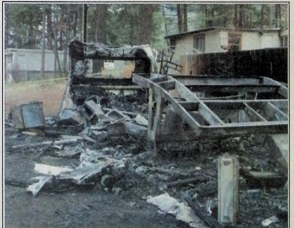
The sleeping occupant of this 5th-wheel trailer in Olalla escaped unharmed thanks to the quick thinking of neighbours around 4:00 AM the morning of November 15th. The trailer was on fire when neighbours awoke and realized someone might still be inside. The heat was so intense they were unable to get close so they threw rocks at the side of the trailer to waken the male occupant.
