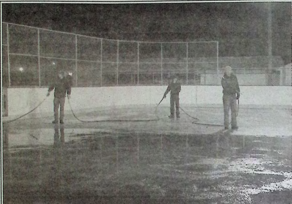
From left, Joe Cottrill, Ivan Gibbs and Keith Erickson of Keremeos started flooding the Keremeos outdoor rink November 27th. With temperatures above zero lately, the refrigeration coils in the rink's surface should keep the rink cold enough to add the required number of ice layers. The ice rink is slated to open the evening of December 7th, coinciding with the annual Keremeos Christmas Light-Up. Photo: Arlene Arlow
