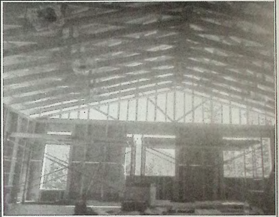
Looking into the shell of the building. Photo: Rob Miller
