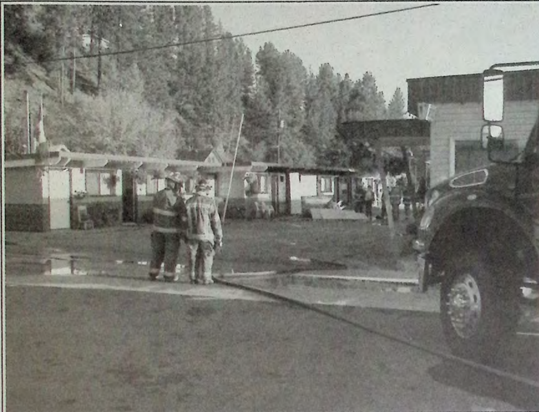
Hours after the early morning fire September 12th at Cedars Motel in Princeton, volunteer firemen were on scene doing mop up and making sure there were no 'hot spots' remaining as a result of the incident. *
