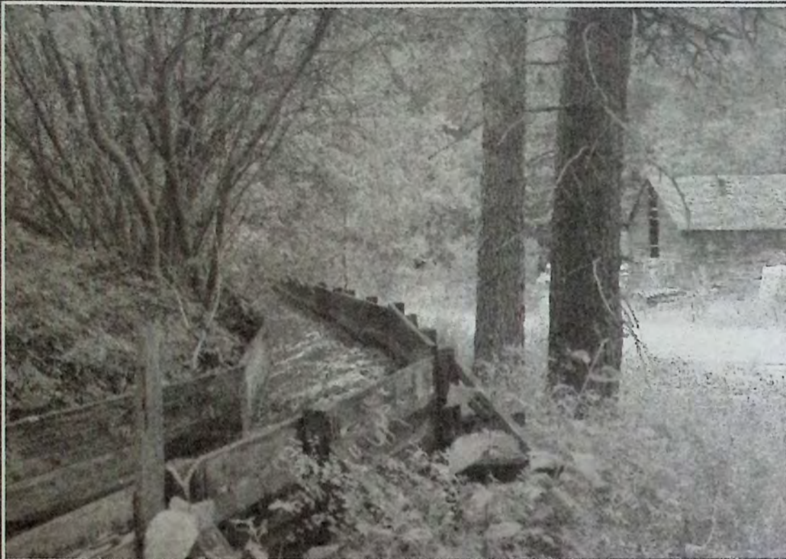
This water flume presents a peaceful picture to those venturesome enough to get out of their cars and climb a 20-foot bank. A mere 50 feet from the Green Mountain Road the water in this flume was running quickly. The old barn in the background adds to the mystique. "I wonder if the wild horses on the Pentiction Indian Reserve use the flume as a watering trough?!" Photo: Arlene Arlow
