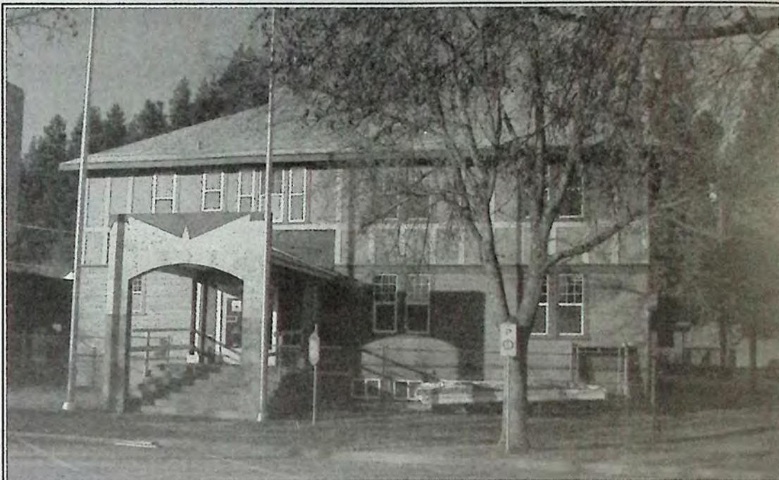
The entrance to the 'new' Town Hall on Vermilion Avenue is just about the last thing to be completed on the outside of the building. Municipal operations moved to the site last week and were operational shortly afterwards. *
