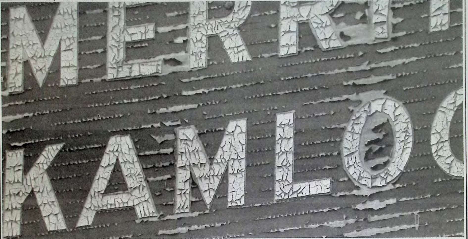
Here's an extreme close up look at the condition of one sign on Highway 3. It needs to be replaced and is apparently on a list for just that. Photo: Brenda Engel
