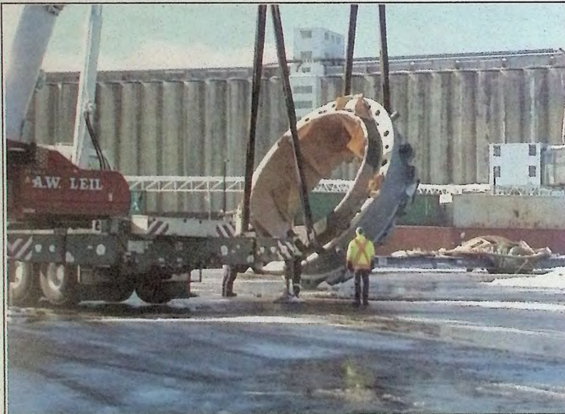
Crews at the Port of Halifax with part of the new secondary crusher which will be used at Copper Mountain Mine near Princeton. The Raptor 2000, once assembled, will be one of just four in the world. - photo submitted
