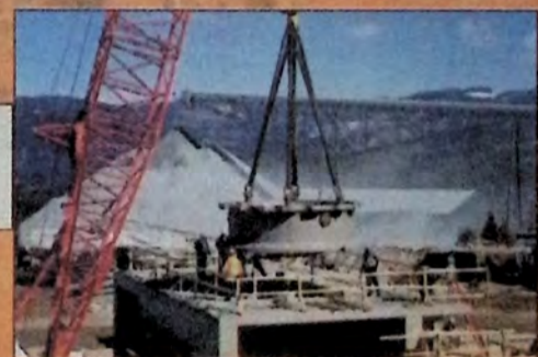
Installation of new secondary crusher to strengthen the future
