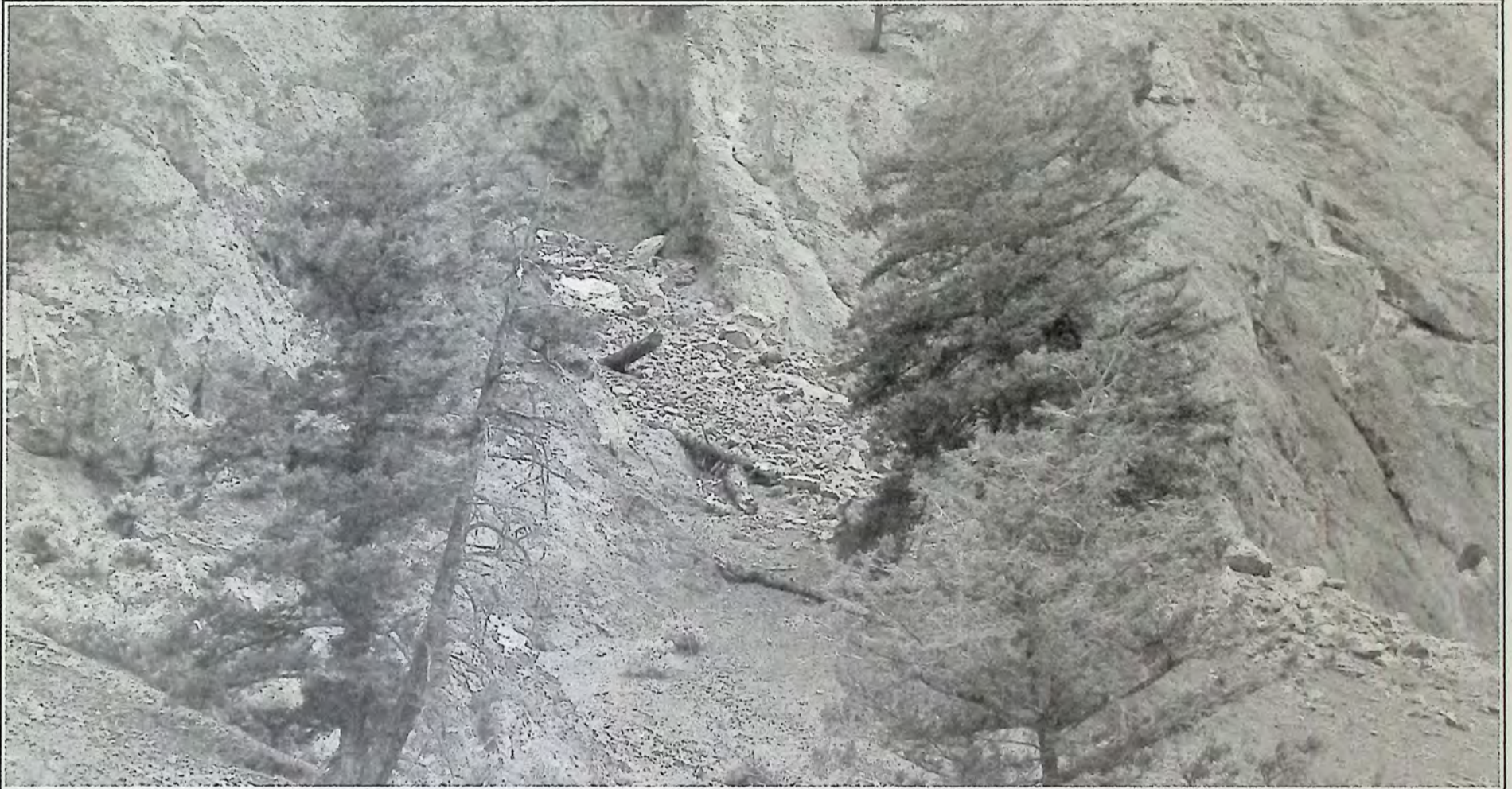
A closer look at some of the new debris that came down the hillside and forced a closure of Highway 3 near Keremeos late in the evening of May 4th. Photo: Brenda Engel
