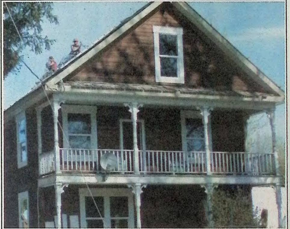
A roof replacement provided a quick update to the classic building.
