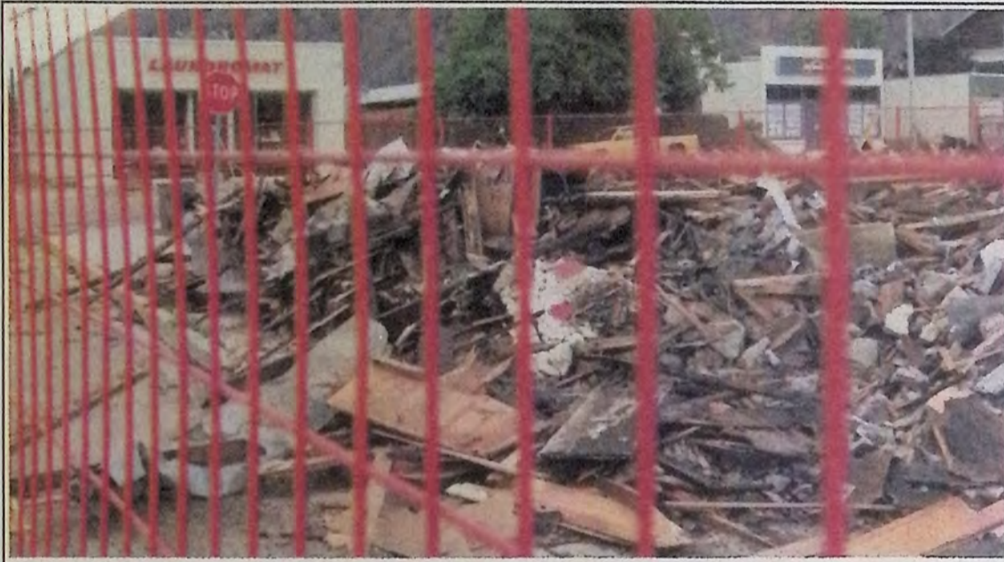
Security fencing surrounds the scene of the recent fire that destroyed the K-Mountain Inn in Keremeos. Although partially obscured the "STOP" sign at the corner of 7th Street and Veteran's Avenue remains in effect. Several kegs of beer and other liquor products were apparently pilfered from the site prior to the installation of security fencing. The debris from the destroyed building will likely need to be inspected for asbestos: asbestos was commonly used in building construction and renovation from the 1950's through to the 1970's. Photo: Arlene Arlow
