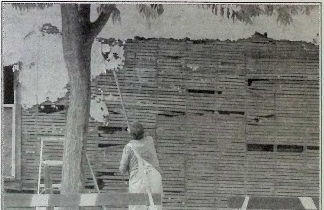
Clean up work and renovations of the former Keremeos Hardware building revealed this interesting exterior during the afternoon of September 29th. This wood was hidden under a layer of plaster board. Photo: Brenda Engel
