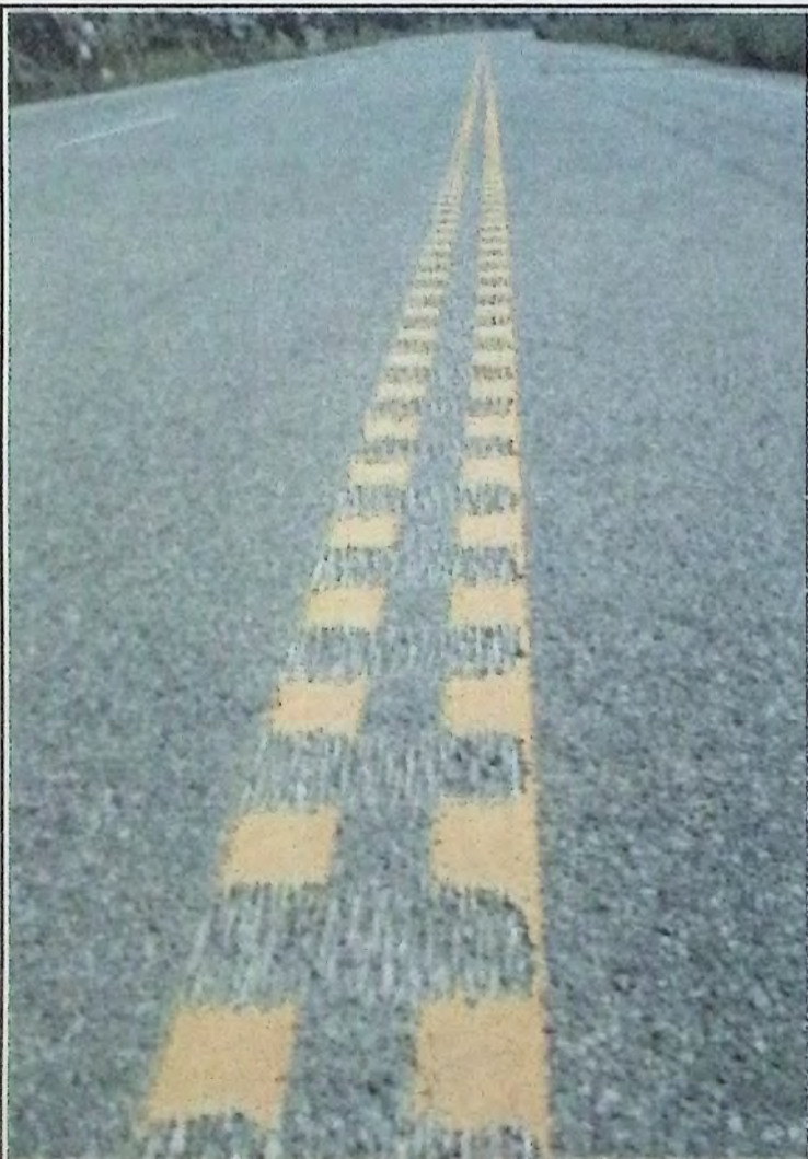
Centre line rumble strips are becoming more common on highways throughout British Columbia as a safety measure. - photo submitted
