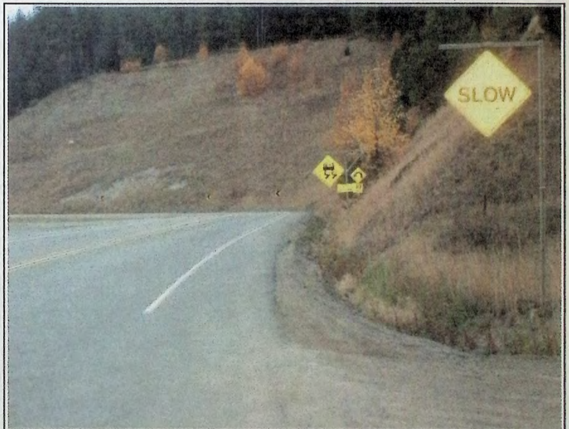
Another high risk area identified along the Hope-Princeton Highway was the approach to Whipsaw Creek Bridge. Additional speed warning signs were installed as one of the educational tools used by ICBC. - photo submitted
