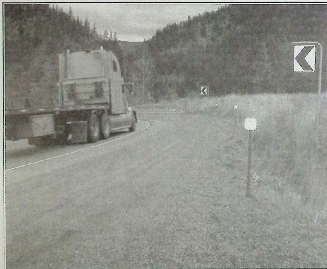
Delineation on high risk corners have been one of many improvements conducted on Highway 3 recently.
