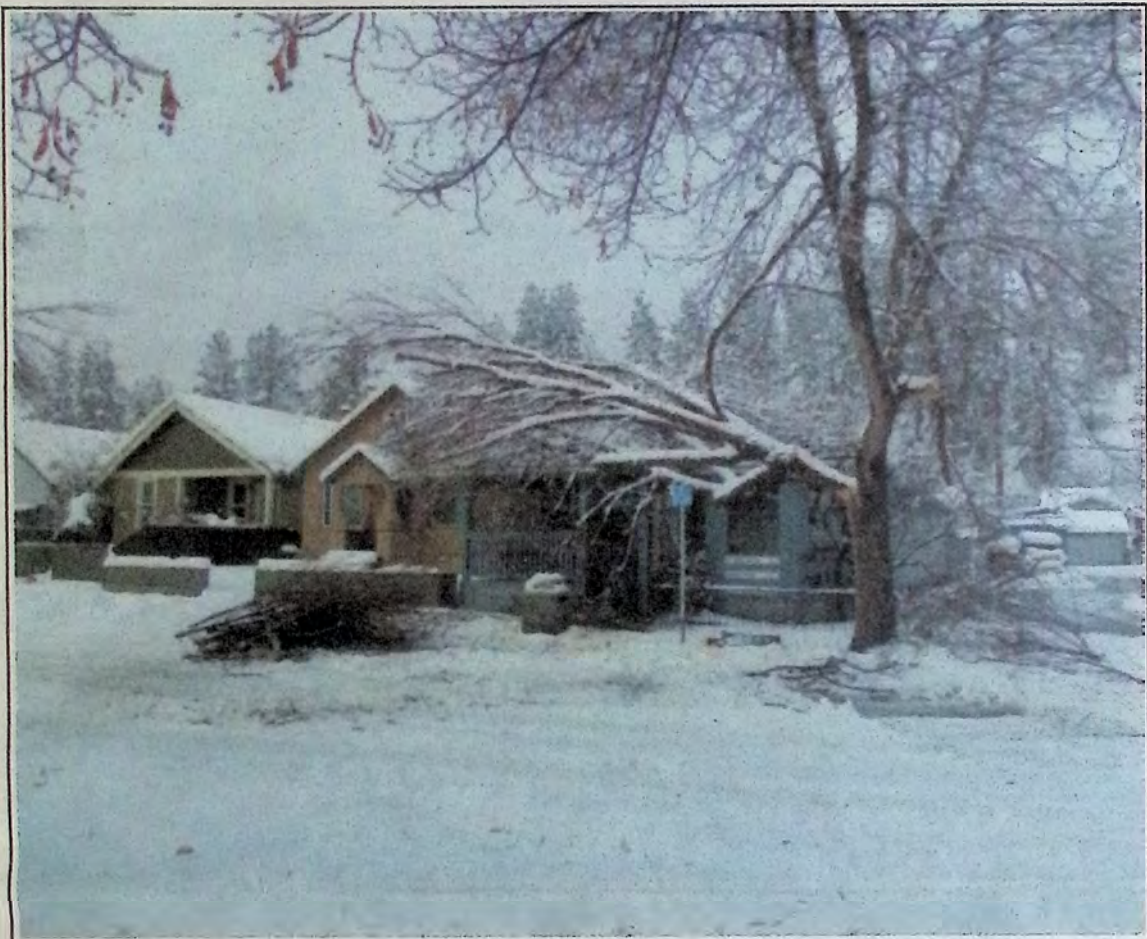
By the time the Town of Princeton Public Works Crew got to this tree they had already cleared away the majority of the serious damage. Tree branches snapped under the weight of wet, heavy snow knocking out power to much of the community and turning downtown Princeton into a ghost town for most of last Wednesday, November 26th. *
