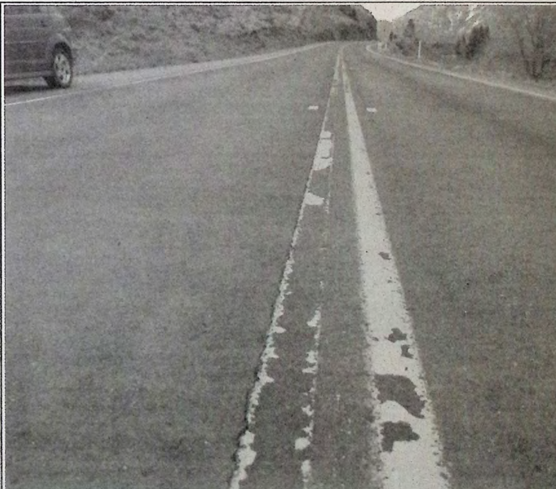
Once upon a time, highway lines were painted with an oil-based paint. The lines seemed to last longer. With the advent of environmental awareness, the Province of BC moved to a water-based latex paint for highway lines. The cost is about 20 cents a metre. The double line in this photo was painted in the summer of 2014. Six months later almost half of the paint is worn off from this stretch of Highway 3 east of Cawston. Much like highways throughout the province, it will stay this way for another few months. The options? Cold plastic costs $10 per metre. And Thermalplastic lines cost $20 per metre. Photo: Arlene Arlow
