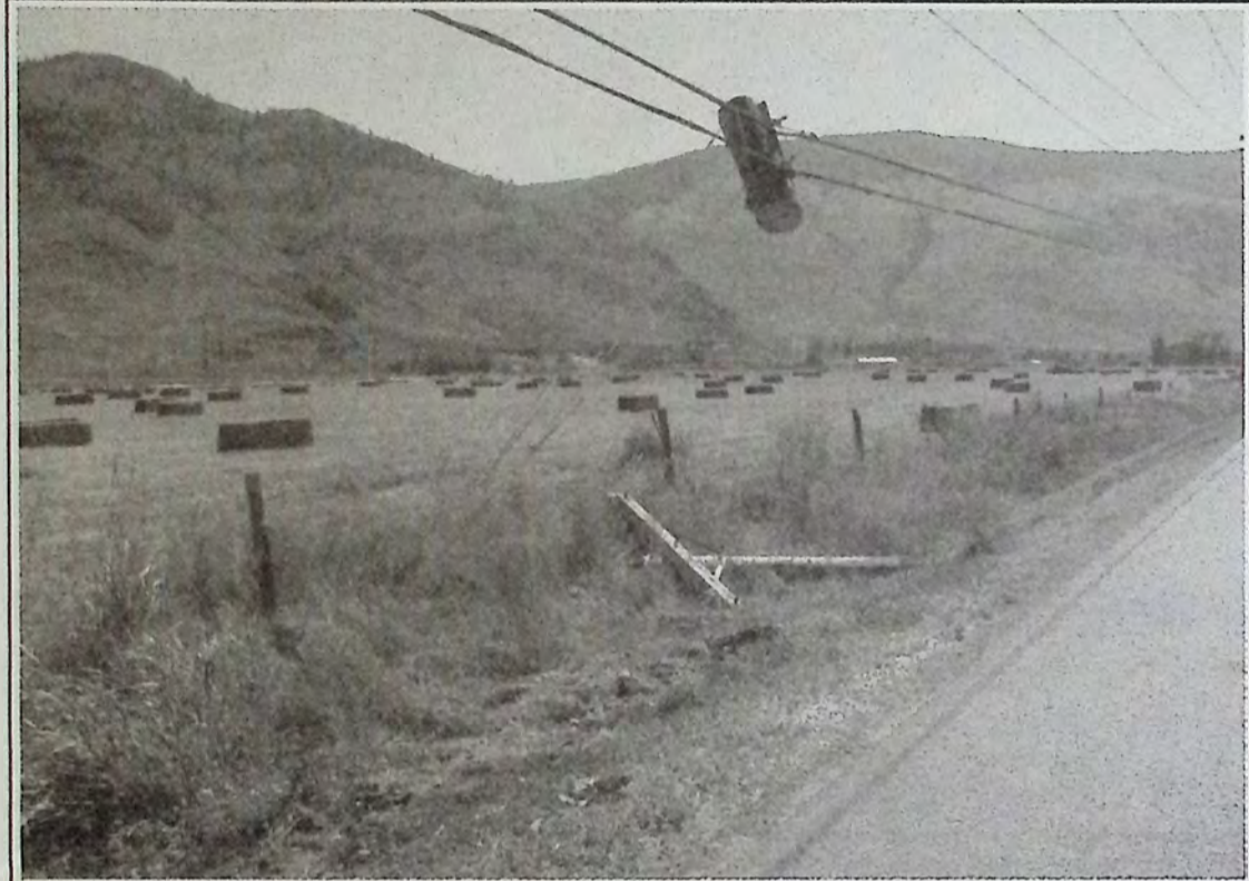
Driving by this scene June 10th on Highway 3 near Cawston caused us to turn back and take a closer look. Yup, a telephone pole is in the ditch and a temporary brace was in place until the pole gets replaced. *
