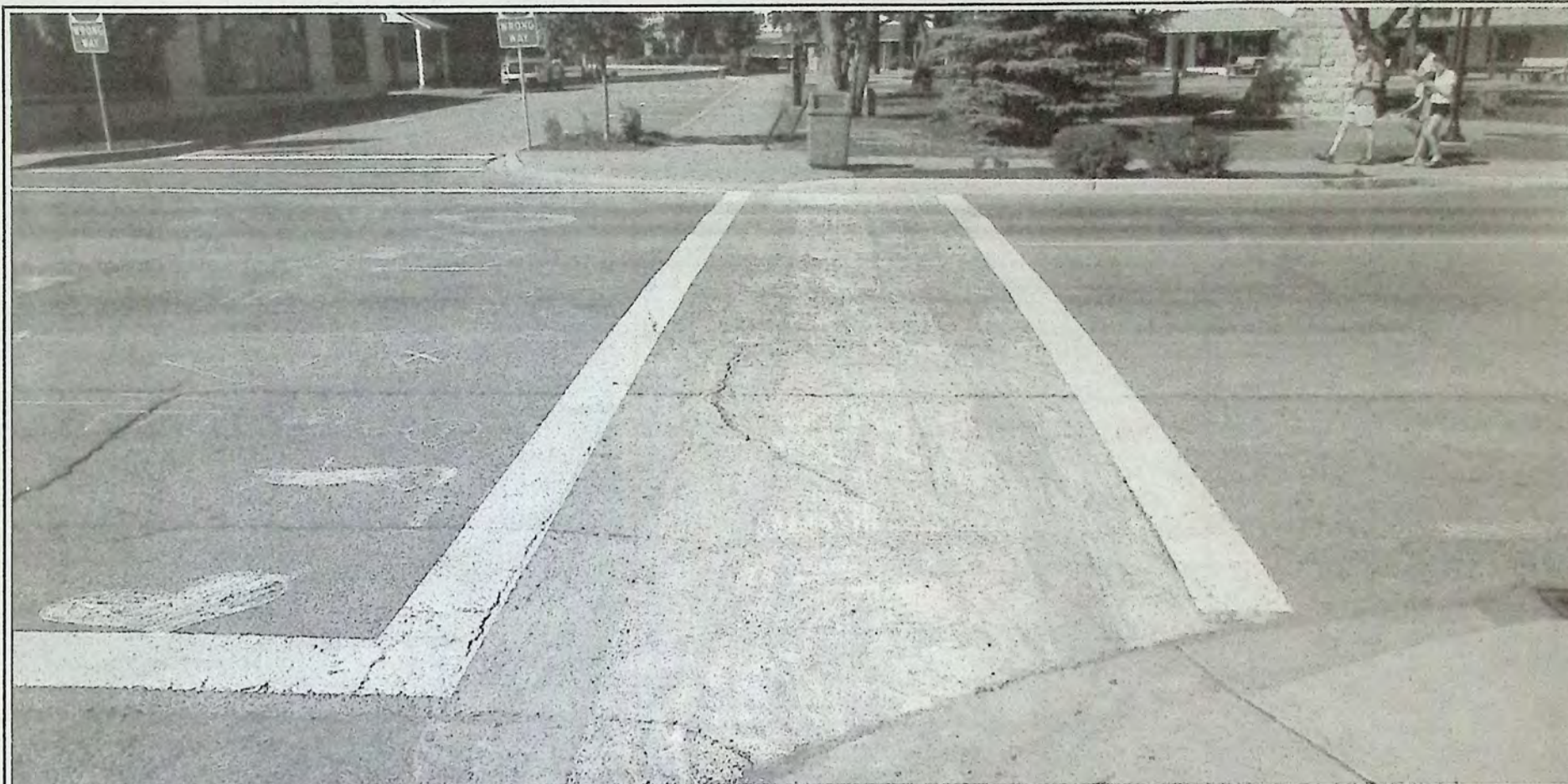
This crosswalk was converted a month ago to a chalk rainbow. Town Council has chosen to make it permanent. *
