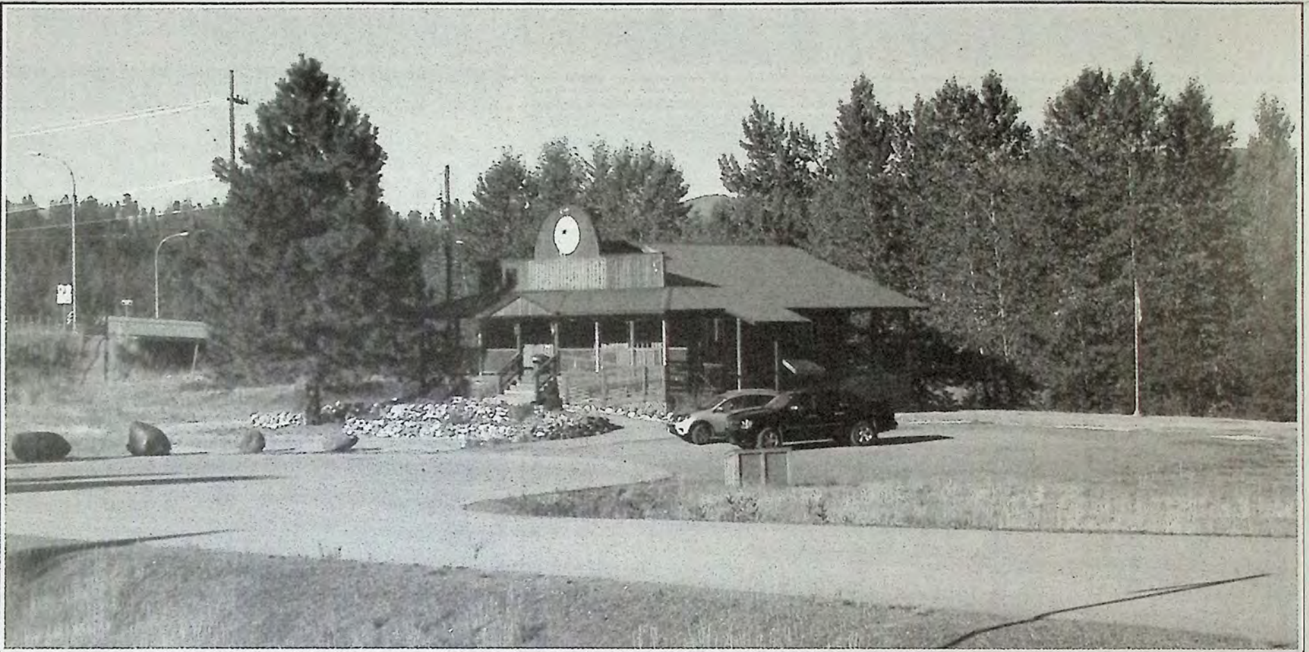
With over 2,200 square feet of living space, this beauty sits on the side of the Similkameen River and has a major highway passing by the front entrance. *
