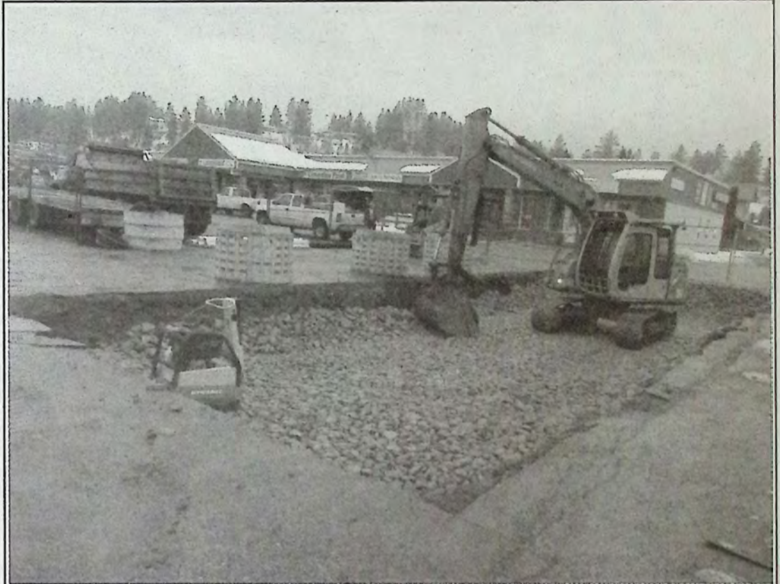
Our 'laugh of the week' comes from contractor Mike Grgich who spent part of last week working on this drainage project at the Princeton Plaza. He jokingly told our photographer he was starting work on the Princeton Pool Project. He said we could quote him on that, so thanks, Mike! We appreciate your good natured humour. Photo: Brenda Engel
