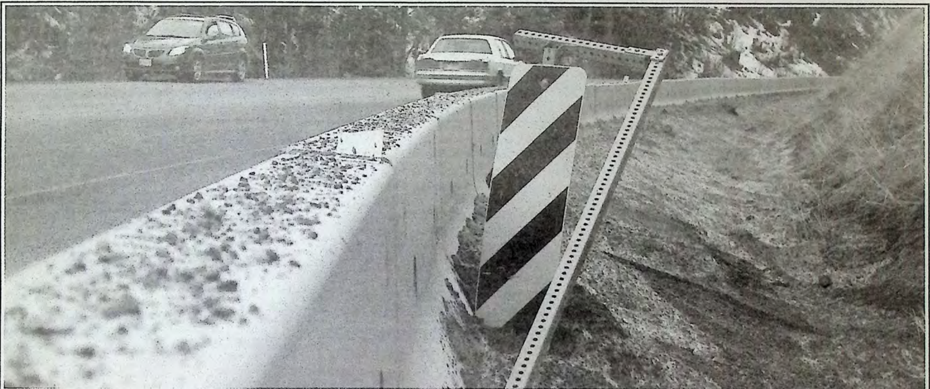
"Nope, it's not workin' for me...". This displaced highway marker westbound near Yellow Lake serves to mark the spot where the snowplow tore it from its moorings. One wonders why these reflective markers are put onto the topside of a cement "Jersey Barrier" instead of putting them further back and suspending them "toward" the road so that drivers can see them - and so that the snowplow blade doesn't trash them. Now that we've got your attention, there is indeed three different kinds of hazard markers on BC highways. Most of us subconsciously know what they mean, but I'll bet if you saw two of them side-by-side on a shelf you wouldn't know left from right. On a highway it is obvious to see what their purpose is. If you see this vertical ^ symbol with alternating bands of black and yellow it means stay to the left or right. This vertical / with alternating bands of black and yellow means stay to the left. And, of course, this vertical symbol \ with alternating bands of black and yellow (you got it) means stay to the right. Your newfound knowledge is relevant, of course, if the sign isn't lying in the ditch. Photo: Arlene Arlow
