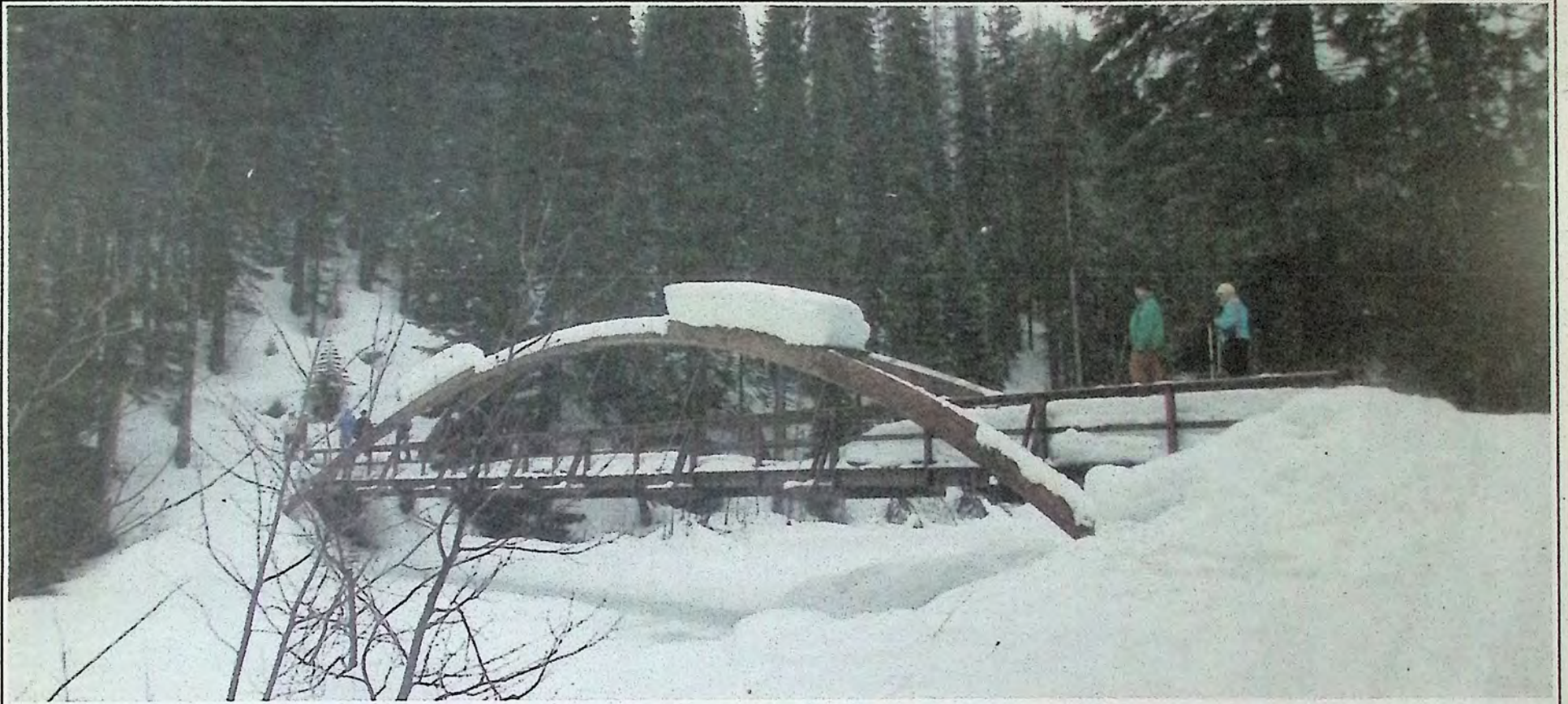
Crossing the Rainbow Bridge at Lightning Lake in Manning Park. Photo: Janis Wright
