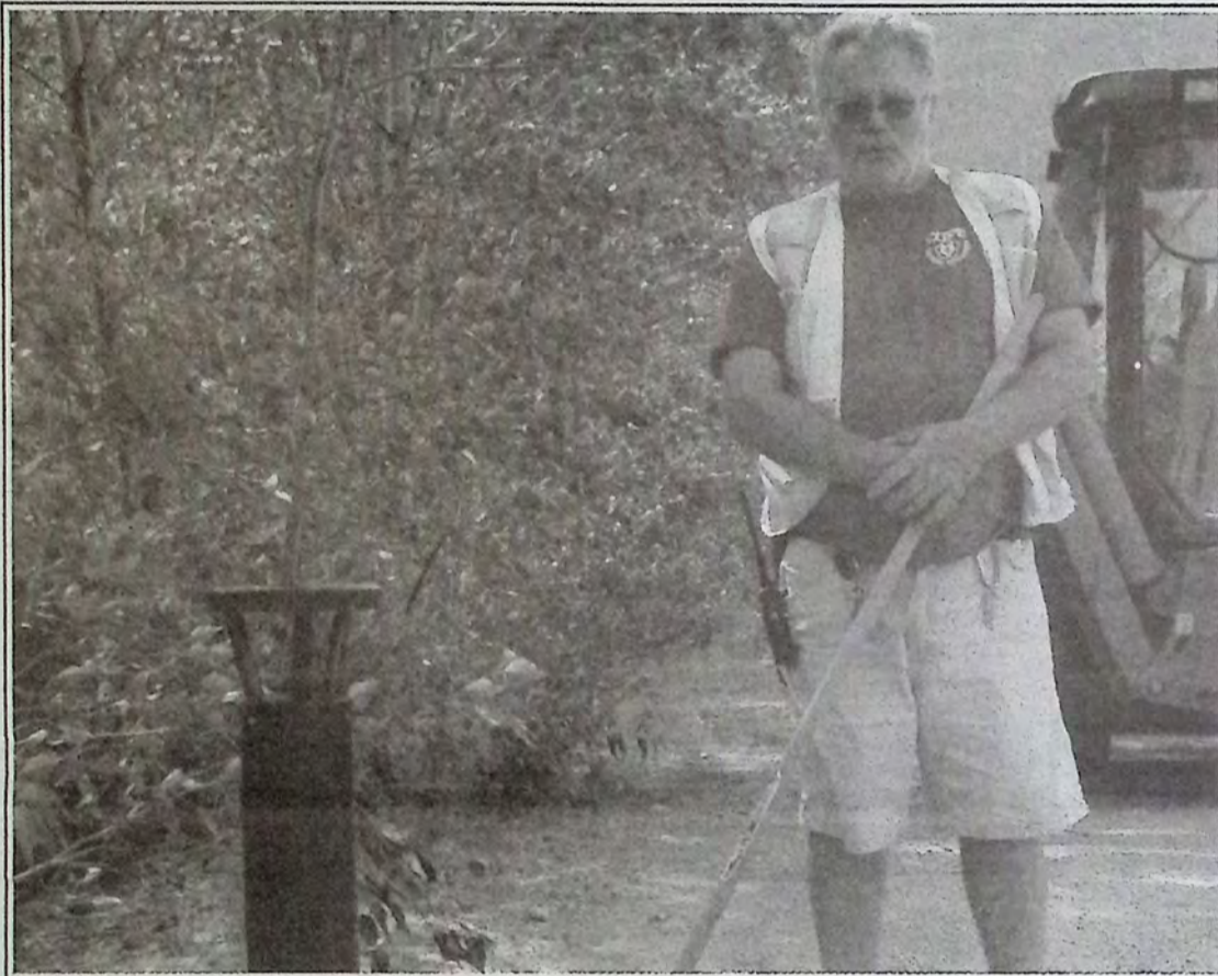
Village crews were recently out putting the spit and polish onto the new Solar Bollards strategically placed around the village. There are 12 on the dyke and four on the Village Promenade. Photo: Marty Menzies
