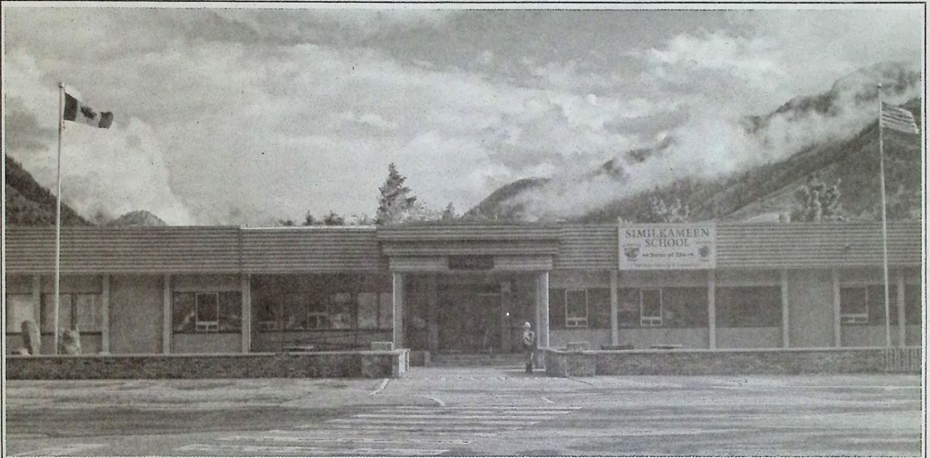
Similkameen Elementary Secondary School (SESS) in Keremeos will receive a major upgrade thanks to the Province of BC. Photo: Marty Menzies
