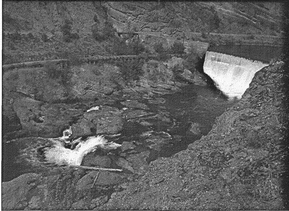
Figure 3.5: Enloe Dam at Squantlen Falls
