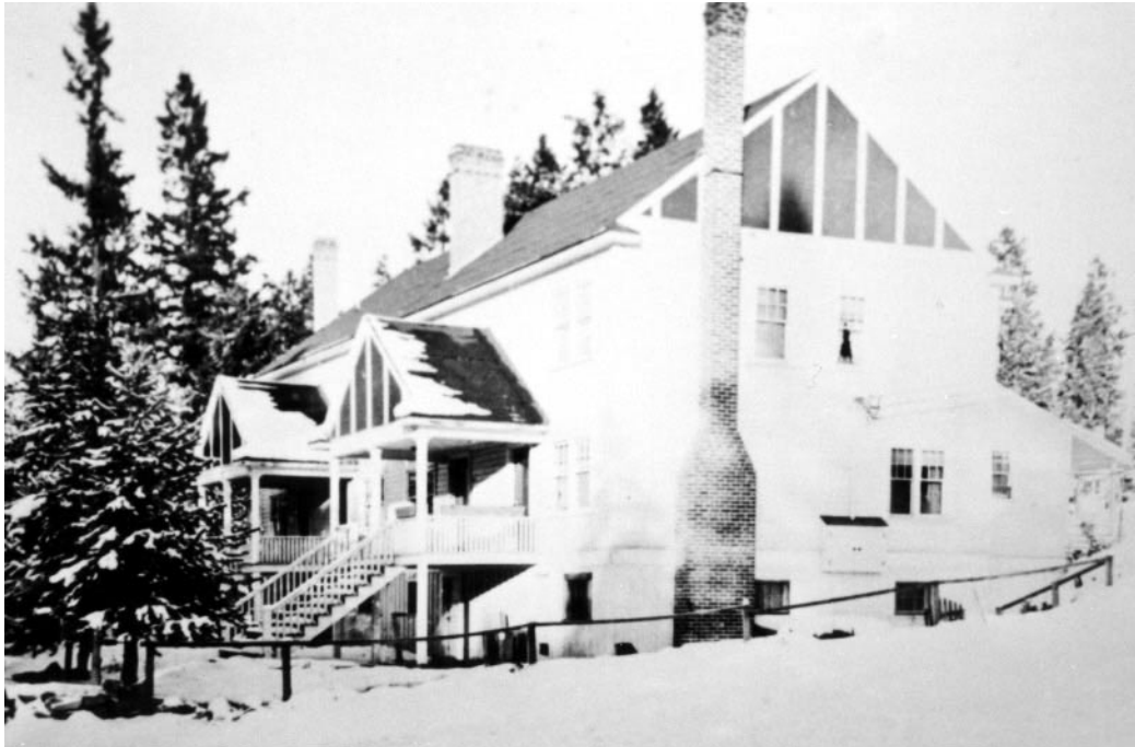
The apartments - 4plex
