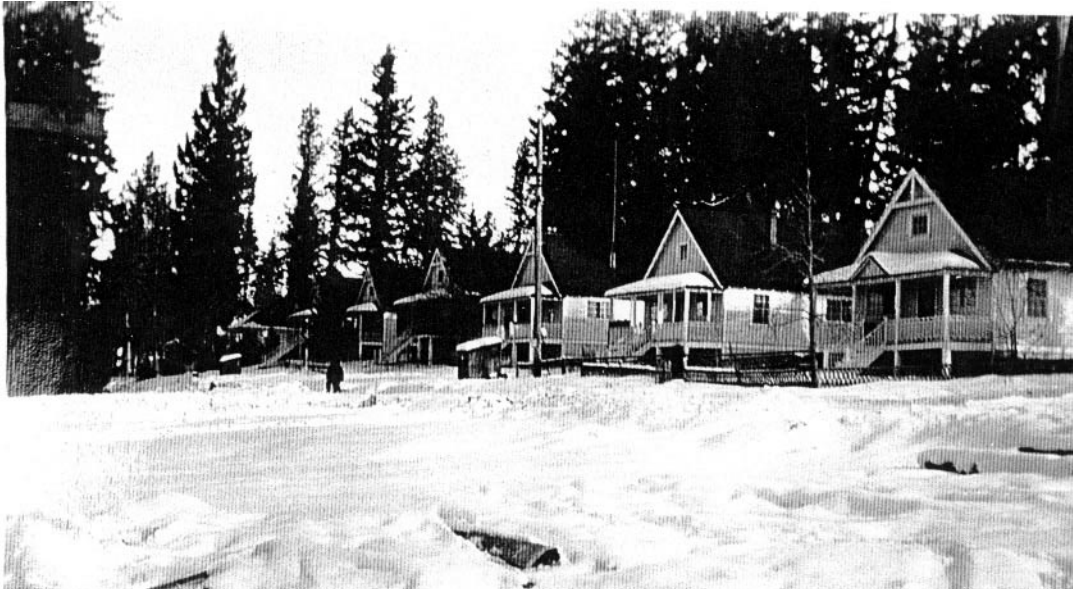
South Town site
